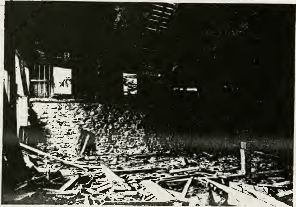
Figure 102. Revenue Mill (structure #34) interior - upper level - north end, east view.
